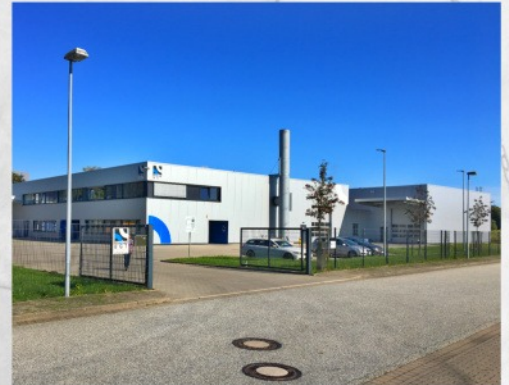
Cordes plant at Boizenburg/Elbe
